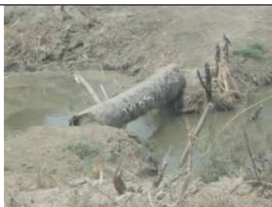
Figure 33: Obstructions through Illegal Bridge at RD 87+007 of Patoyun Br Drain
