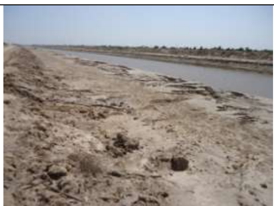
Figure 45: Damaged Berm and Bank of Spinal Drain RD 578
