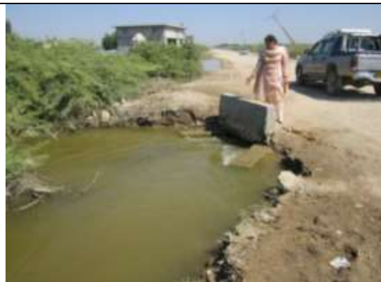
Figure 17: Inadequate Capacity of Road Culvert Nawabshah Component
