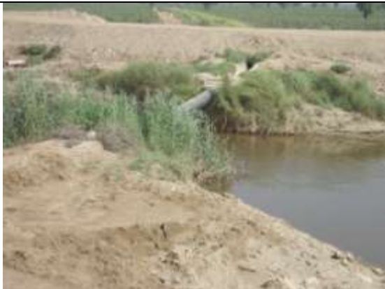
Figure 20: Illegal Pipe Crossing at RD 11+498 of WNMD
