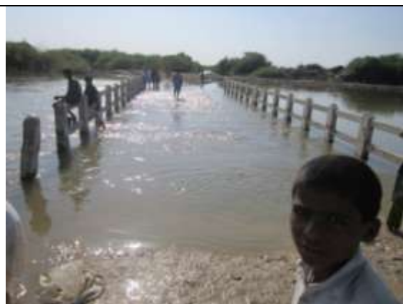
Figure 42: Overtopping of LBOD Branch Drain at Outfall point RD 203 Spinal Drain
