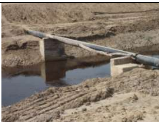
Figure 23: Illegal Pipe Crossing of WNMD 49
