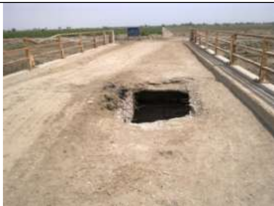
Figure 28: Damaged VRB at RD 132+460 of Sinjhor Br Drain
