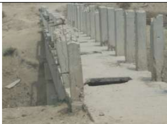
Figure 31: Damaged WCA at RD 70+069 of Patoyun Br Drain
