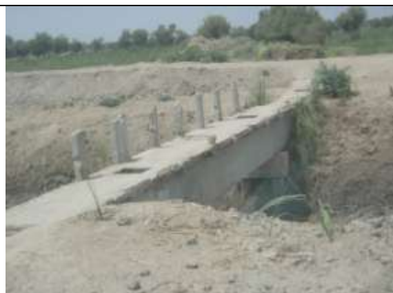
Figure 30: Damaged Foot Bridge at RD 42+000 of Patoyun Br Drain
